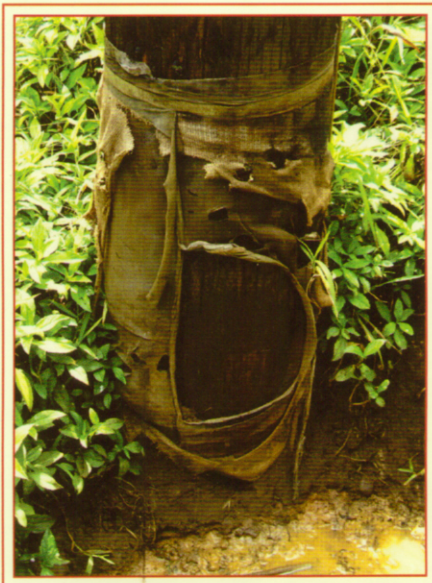
Feral pigs have damaged a mesh sock above ground.
